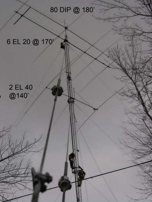
80M #2 Dipole at 180' 40M #2 2L at 140' Upgrade to 2L/2L W6NL Moxon design
